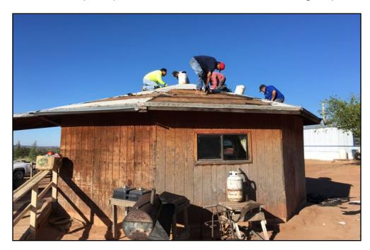
t e m p o r a r y employees to begin working on repairing the roof of the hogan. The team quickly stripped the roof, but had to wait f o r s o m e a d d i t i o n a l supplies to arrive before they could repair the fascia boards and begin
