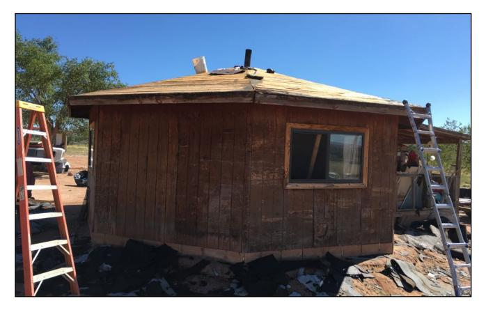
laying down felt paper. The team worked all day in the searing heat and by the end of the day, had completed the felt paper installation and began installing shingles.
