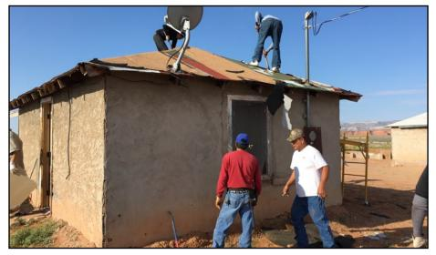
members from OPVP and Department of Transportation, the repair work was done. These repairs included removing the roofing materials and replacing with new felt and roofing paper, replacing drywall, painting, and replacing floor tiles.
