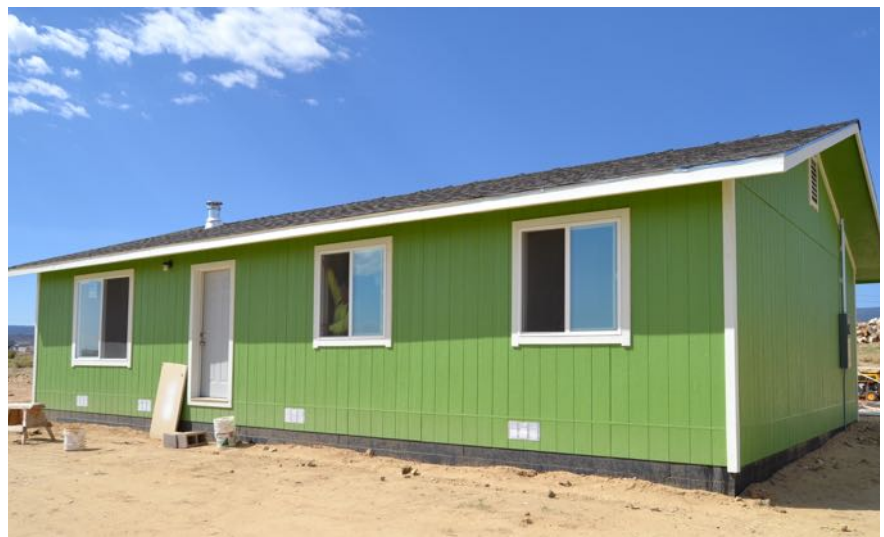
Naschitti Complete-Build Project Site
