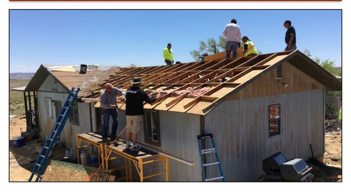
On Friday, May 5, the DCD Team gathered at a veteran's house in Twin Lakes and began tearing off the old tattered roofing paper and rotting plywood to put on a new layer of roof underlayment to give the roof stability. The team then applied new roofing paper and began installing new shingles. The day was hot but some occasional clouds and a slight breeze provided a refreshing relief. The team moved at a good pace and before long, the most damaged wing of the house had been repaired.
