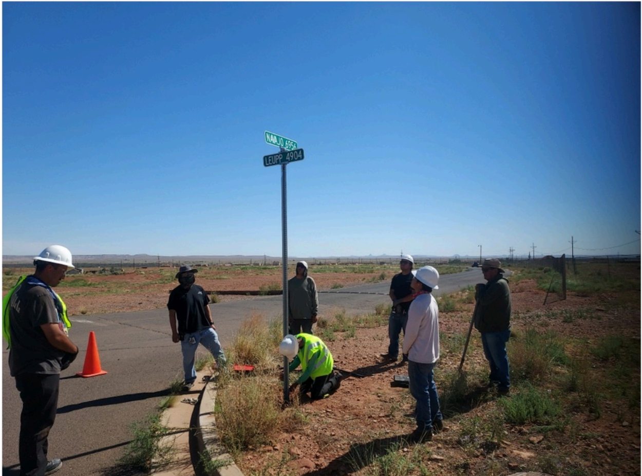
Leupp laborers installing an intersection sign on Leupp School Incorporated campus
