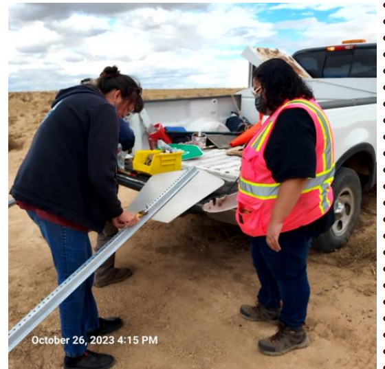
Ms. Michele Peterson, Shiprock Chapter Manager, and Jessica Johnson, Shiprock LRAC, are fastening a sign shield to the U-channel base post with tamper-proof nuts north of Shiprock Chapter; the sign will be installed onto a 40" base post that has already been installed and 4" is sticking out of the ground
