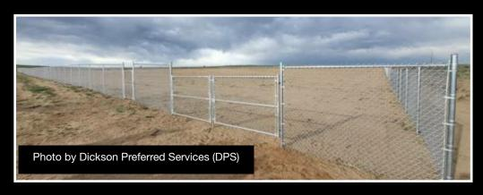
Phase 1 of the project was successfully completed in June 2023. This phase involved leveling the cemetery grounds and constructing a commercial-grade 6 ft chain link fence around the 10-acre cemetery perimeter. The result was a well-prepared and secure space for burials.
