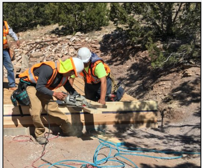
CONSTRUCTION WORKERS BUILDING A BATHROOM ADDITION
