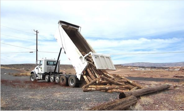
Joe Dirt Excavating delivers wood at the Cameron Chapter House March 6. The delivery is part of a pilot project by the National Forest Foundation, U.S. Forest Service and the Cameron Chapter to provide wood to residents who may not be able to travel to retrieve it from the forests. (Katherine Locke/NHO)
