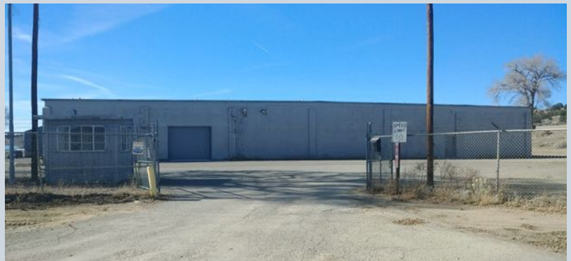
GAMERCO STORAGE SITE (EXTERNAL)
