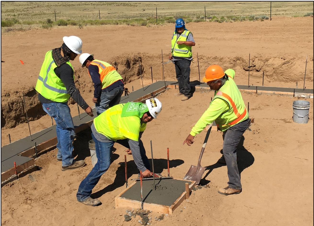
Once the trenching was done, it was time for building the forms for the footings. DCD staff from the Community Housing and Infrastructure Department provided the expert guidance to make sure the team built the forms to exact measurements. Once the forms were in place, a cement truck brought in concrete and poured it into the forms. The crew quickly smoothed out the concrete before it set to form a solid base for the cinder blocks.
